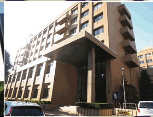
IMR Building 1 (Nojiri Lab., A06)
